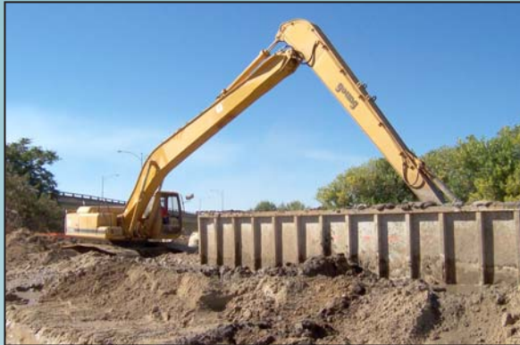
Construction of a slurry cutoff wall
