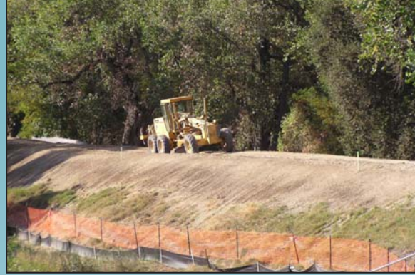
Levee embankment grading
