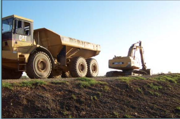
Hauler and excavator on levee crown
