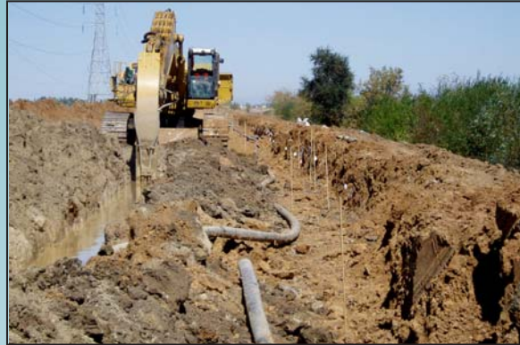
Construction of a slurry cutoff wall
